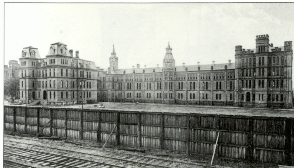
The North Carolina General Assembly in 1869 authorized “a penitentiary with a stockade and buildings to contain 500 cells.” The first prisoners were housed in log cabins on the new prison grounds while an Ohio architect, Levi T. Schofield, designed the permanent building. The first block of sixty-four cells opened in 1875. The original complex, a four-story Gothic Revival brick building, was completed in 1884. The postcard view shows how the prison appeared from West Morgan Street a few years after the turn of the century.
