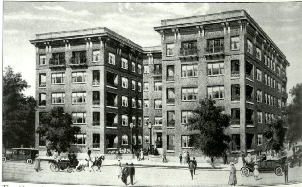
The Capital Apartments, a five-story brick structure, was constructed in 1917 at 127 New Bern Avenue. This is one of Raleigh's earliest "high-rise" apartment buildings and features a U-shaped layout, which allows light and breezes to reach all the apartments. Only a block from Capitol Square, the conveniently located building still is used as an apartment complex.
