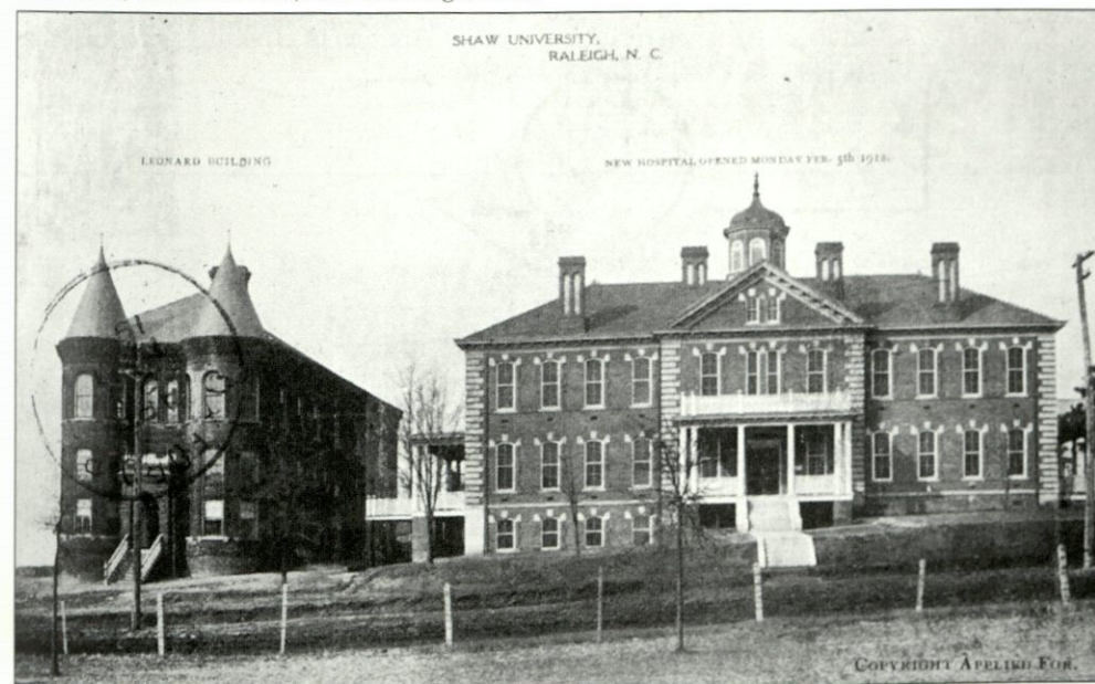
The Leonard Building (left), completed in 1881, housed a medical school "to train Christian physicians to serve the health needs of the Negro Race." Shaw's first hospital, which opened in 1885, was replaced in 1912 by the brick structure shown on the right. The handwritten message on the back of the card, postmarked April 26, 1912, reads, "Does it look natural. Prof. E. designed and constructed it. Wish you could see it. Annie."
