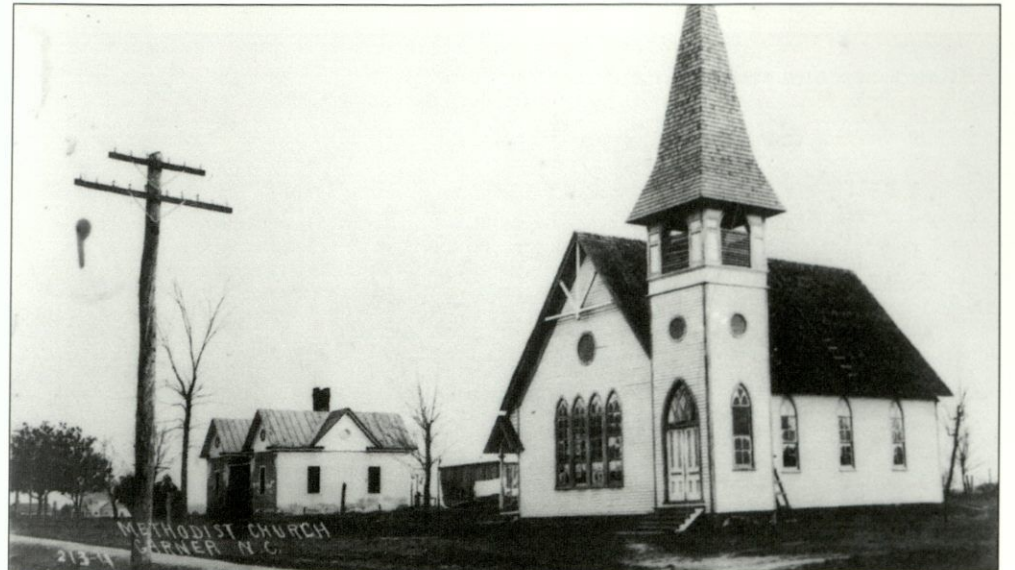
For more than sixty years, the congregation of Garner's Methodist Church worshiped in this building, which was constructed in 1892 on the corner of Main and Griffin Streets. When the Methodist Church moved in 1959 to its new home on Oak Circle, just off Vandora Springs Road, their old church was sold to the Wake Baptist Church. The building, shown here on a real photo card, was taken down in the 1970s. (Kaye Whaley.)
