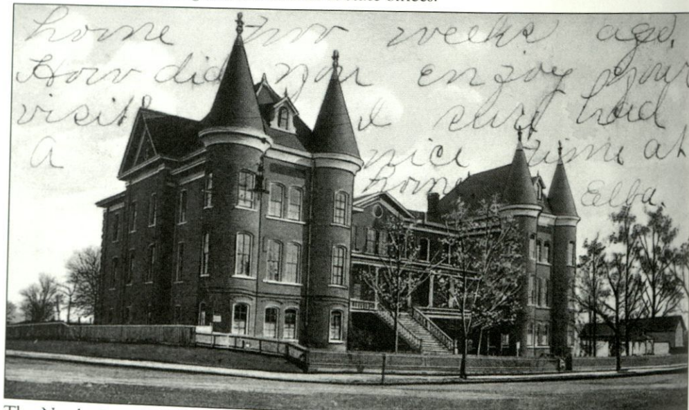
The North Carolina Institution for the Deaf, Dumb and Blind established a department for black children in 1869. The students were housed for the first few years in space rented in the Washington School. In 1874, permanent buildings were erected on a one-acre site bounded by Bloodworth, South, Person, and Lenior Streets. The Raleigh Institute of Cosmetology was the last occupant of the remaining portion of the main building, which was taken down in 1992.
