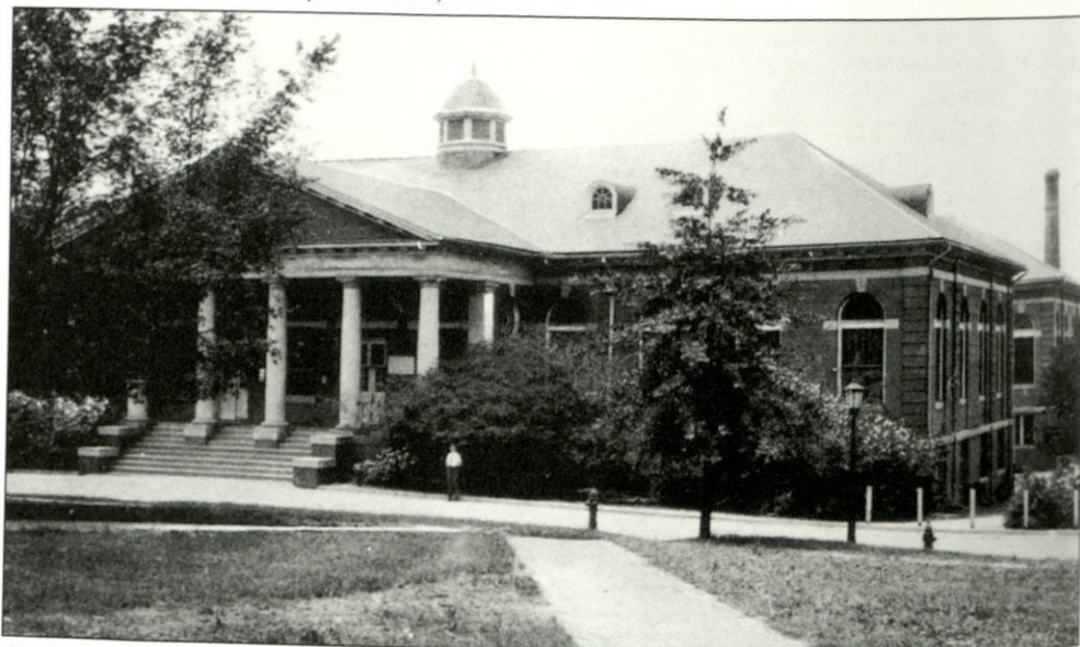
As the student body grew, dining facilities were moved from the Main Building (Holladay Hall) to Watauga Hall, and then to Pullen Hall. Leazar Hall (1912) served as the main campus dining facility until the early 1960s. Located on the south side of the Court of Carolina, Leazar faces the backside of Watauga. The Dairy Records Center, Design School laboratories, and computer laboratories presently occupy most of the building.
