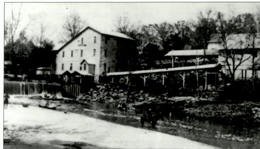
The "Great Falls of the Crabtree" was the site for a succession of mills as early as 1778. In 1908, Cornelius J. Lassiter purchased this mill site and built the gristmill seen here, using two 40-horse turbine wheels to generate power to mill wheat, corn, and later, lumber. Destroyed by fire in 1958, the mill site is still owned by the Lassiter family today. (Courtesy Office of Archives and History, Raleigh.)
