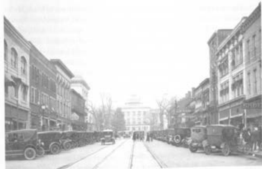
Fayetteville Street looking north toward the Capitol, circa 1920s.
