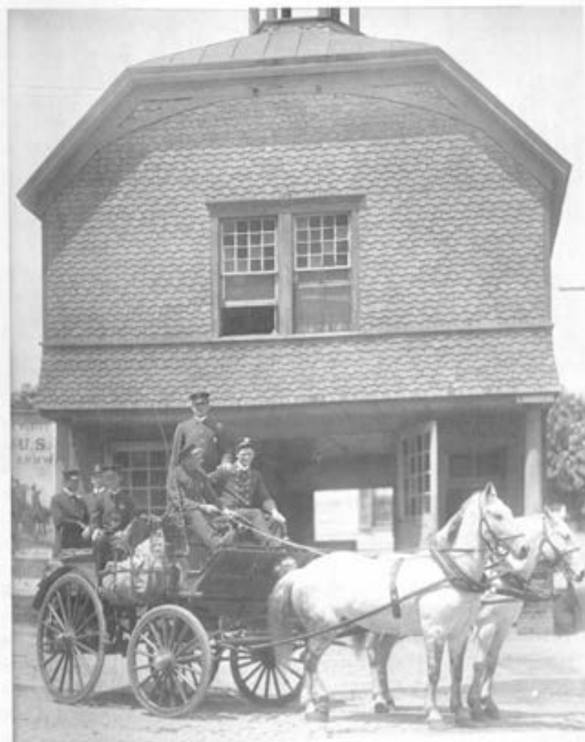
Hook and Ladder Fire Station No. 3, circa 1911-12.
