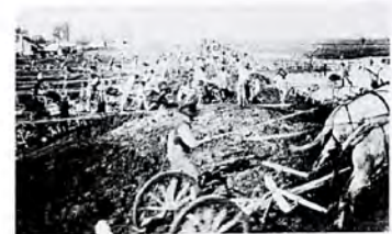
Early levee construction
