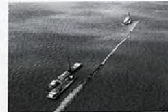
Restoration of jetties in the Southwest Pass [U.S. Army Corps of Engineers]
