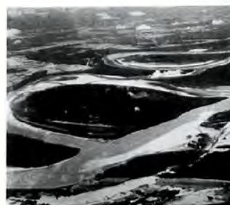
Greenville cutoff, 1930s [U.S. Army Corps of Engineers]
