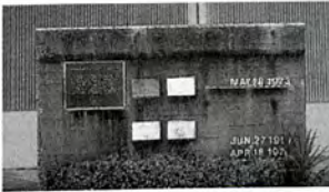
Commemorative marker at the floodwall, Morgan City, Louisiana
