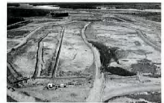
Site of the Old River Control Structures, Simmesport, Louisiana [U.S. Army Corps of Engineers]
