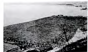
A giant willow mat, a predecessor of today's concrete revetments, being laid in place to prevent bank erosion [U.S. Army Corps of Engineers]
