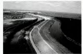
Basin protection levee of the Atchafalaya Floodway
