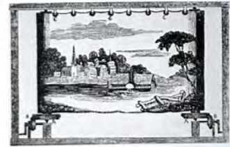
The machinery for John Banvard's Moving Panorama, from Scientific American , December 16, 1848
