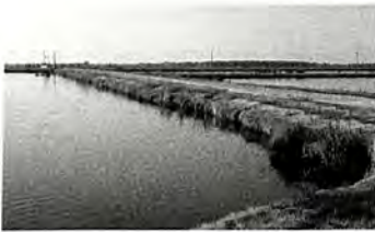
Low levees defining catfish ponds
