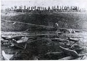
Levee construction, 1800s [U.S. Army Corps of Engineers]
