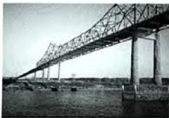
Buoys and bridges frame the shipping channel
