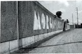
Floodwall, Morgan City
