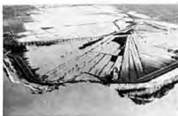
A growing crevasse on the River Road [U.S. Army Corps of Engineers]
