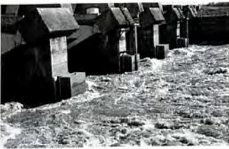
The turbulent discharge at the Auxiliary Control Structure
