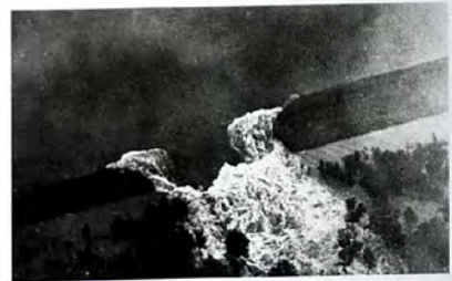
A levee break in the Great Flood of 1927 that submerged 23,000 square miles from Cairo, Illinois, to the Gulf of Mexico, reportedly destroying more than 160,000 homes and killing between 250 and 500 people [U.S. Army Corps of Engineers]
