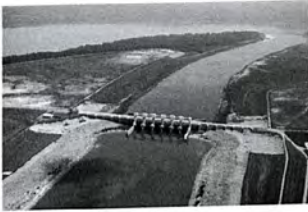
The Auxiliary Control Structure [U.S. Army Corps of Engineers]
